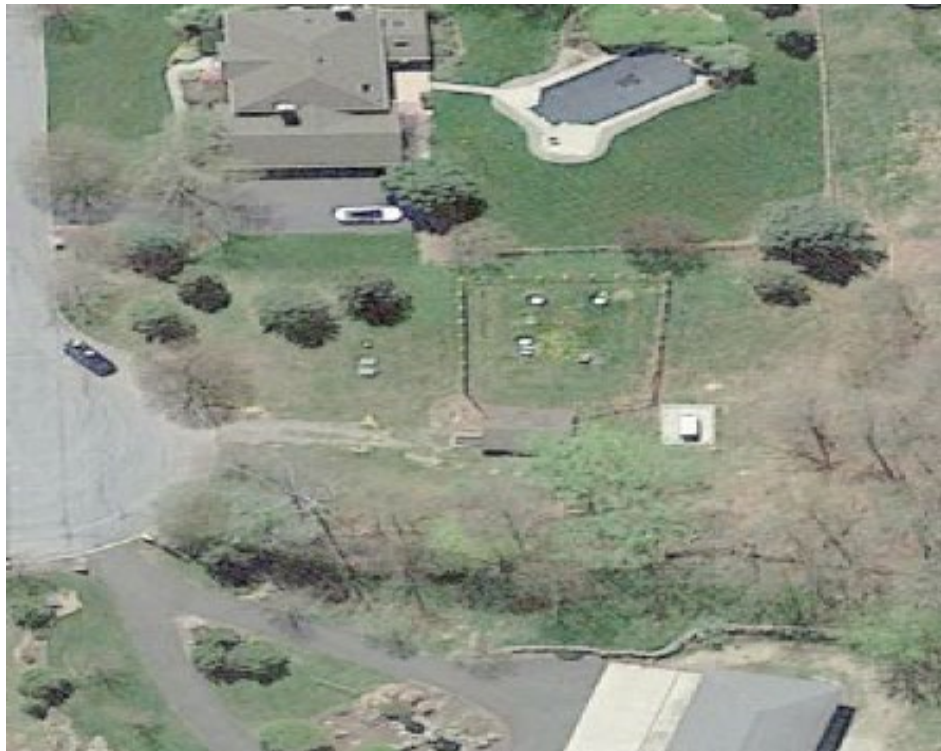
AERIAL VIEW OF PUMP STATION SITE
