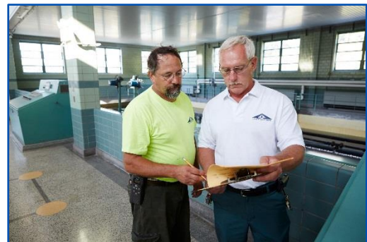
Water Filtration Plant Filter Beds / Underdrains - Installed 1958 To be replaced 2019-2020 - $13M
